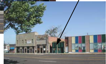
3,348 sq. ft. of land available behind the facade
